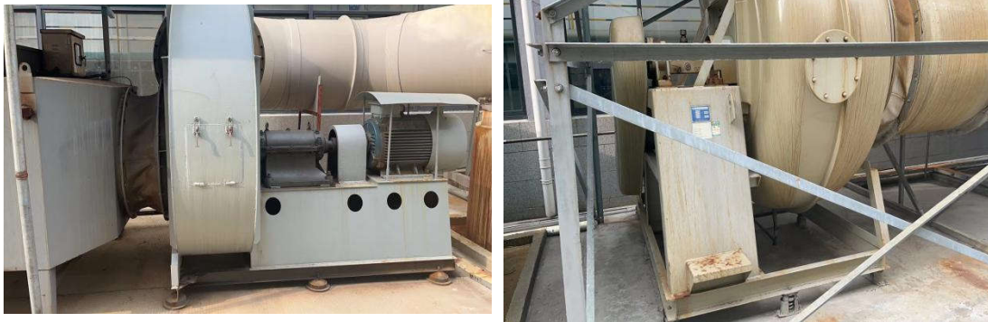
风机加装减振地脚及防护外壳
