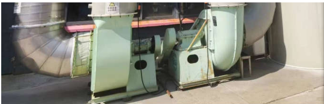
风机加装减振地脚及防护外壳
